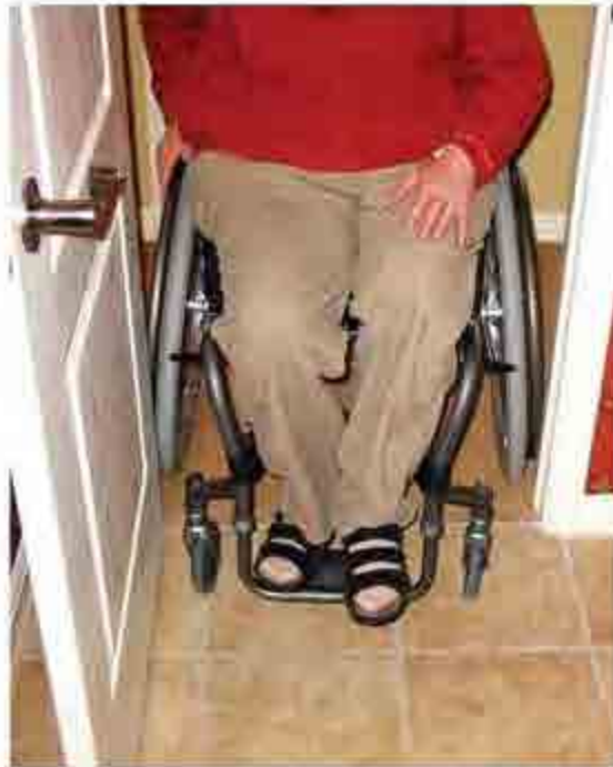
28" doors block entry to wheelchair users
