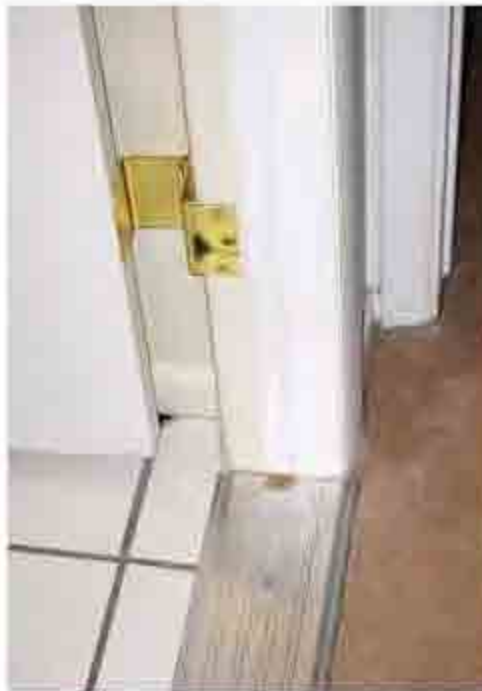
For retrofits, 30" doors on swing clear hinges allow passage for most wheelchairs
