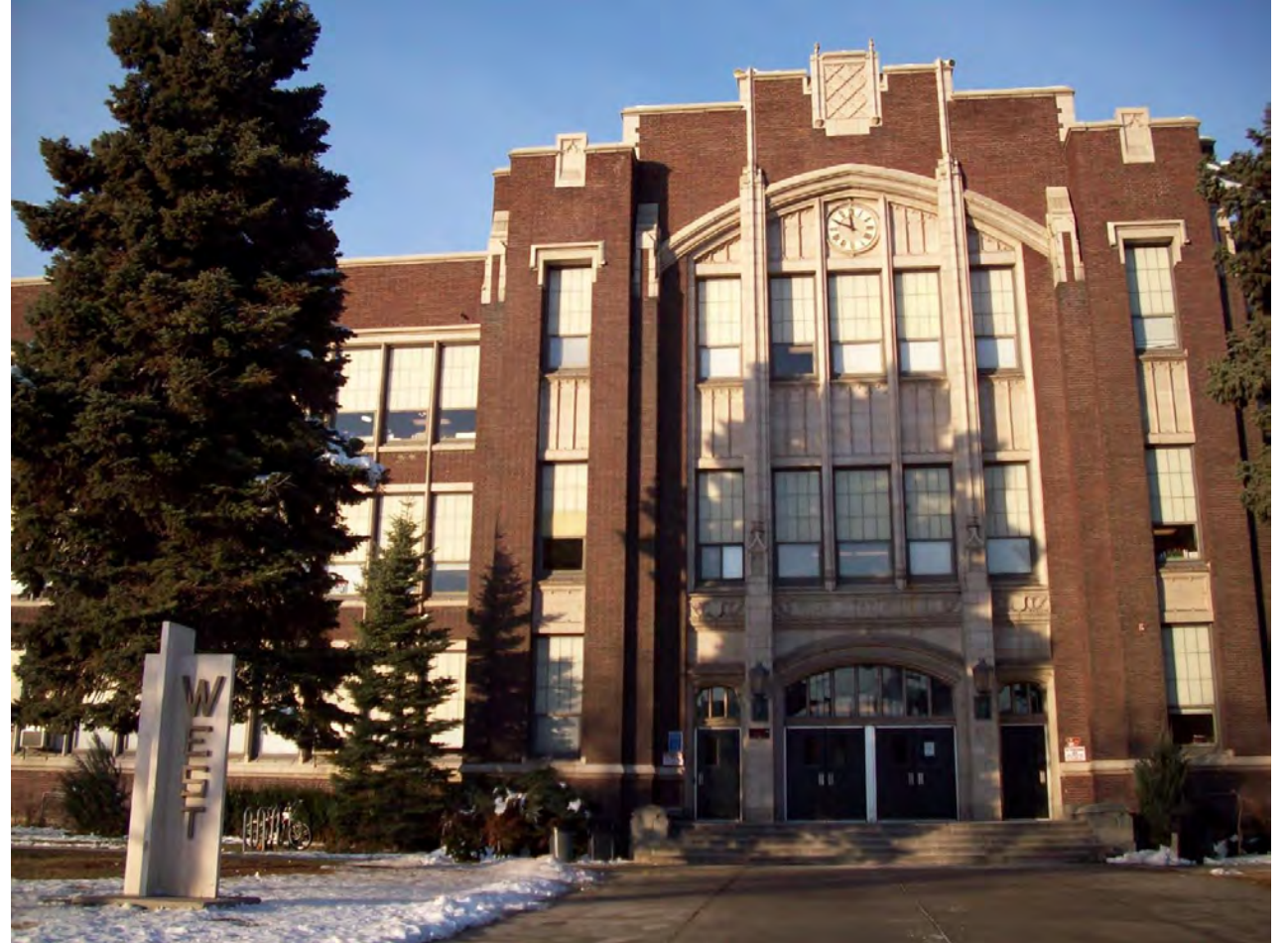
WEST HIGH SCHOOL IS A URM SCHOOL THAT WAS RETROFITTED IN 1996.
